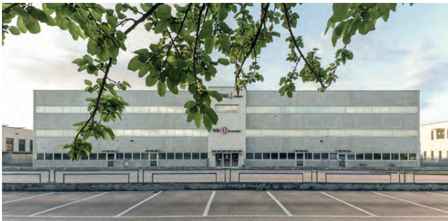
BTK Headquarters - NORTH ITALY
